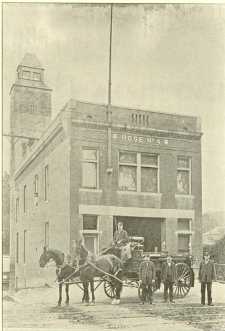
FIRE HALL NO. 4. Third and Franklin Streets.
